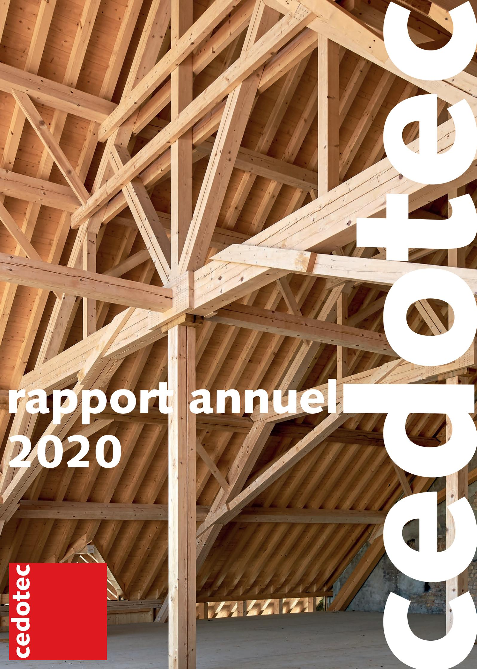
A detailed view of a wooden roof truss structure, showing a complex network of light-colored wooden beams and rafters. The structure is supported by a central vertical post. The lighting is warm, highlighting the natural grain of the wood.
